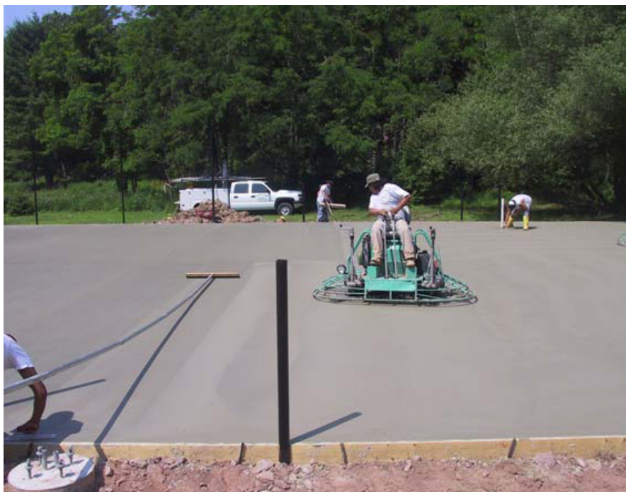
Figure 2. The concrete finishing “Zamboni” slides over setting concrete.
