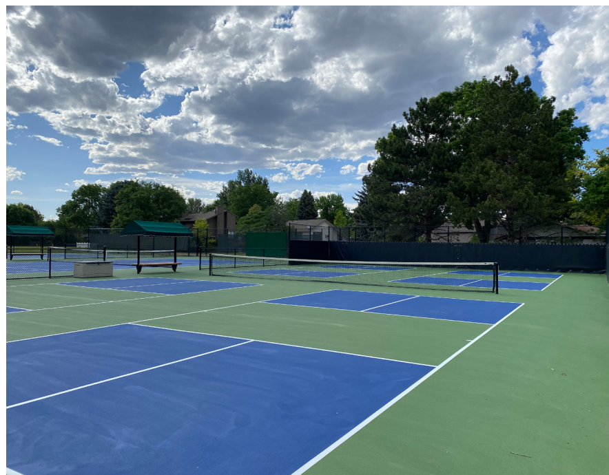
Figure 3. Acoustifence installed inside pickleball court fencing. A bit of reverb has been noted inside the Acoustifence enclosure.
